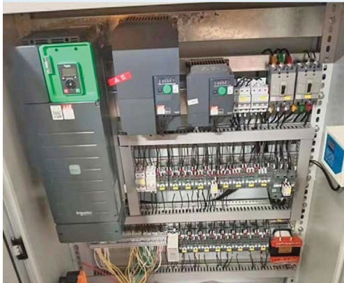
Crane & Hoist VFD Modernization Panels
